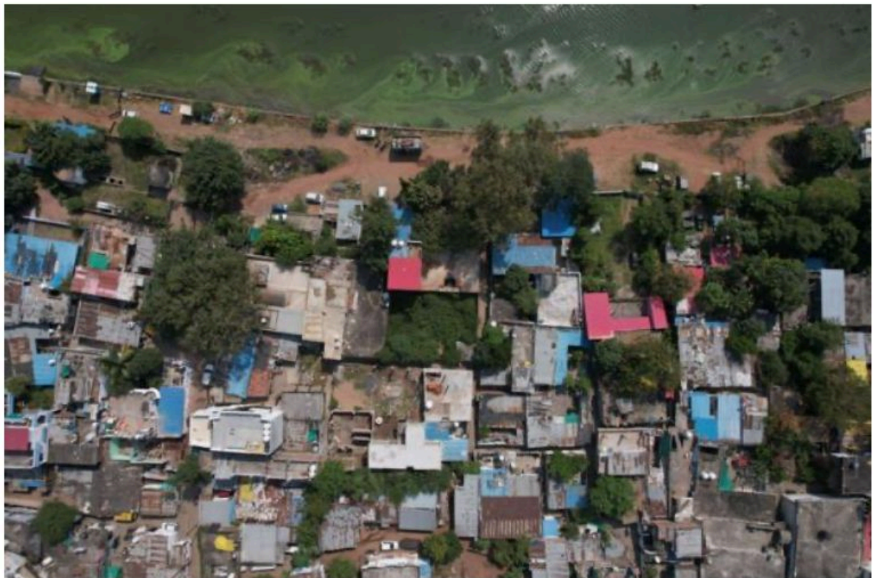
Figure 13: The Khanu Gaon settlement and the protective retaining wall constructed at its periphery to prevent water from entering the settlements
