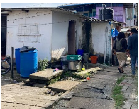
Concrete slabs over drainage channels
