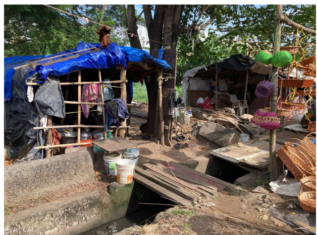
Kutchra houses near open drain
