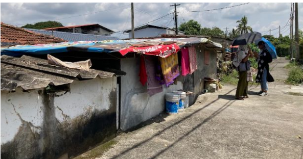
Older homes with cement sheet roofs covered with plastic sheets
