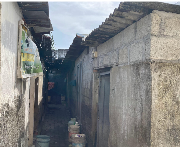
Newly constructed houses made of concrete blocks with cement sheet roofs.
