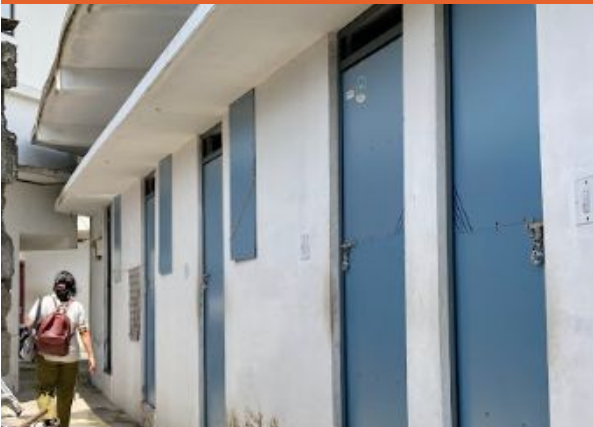
Single-room units constructed specifically for renting to migrants
