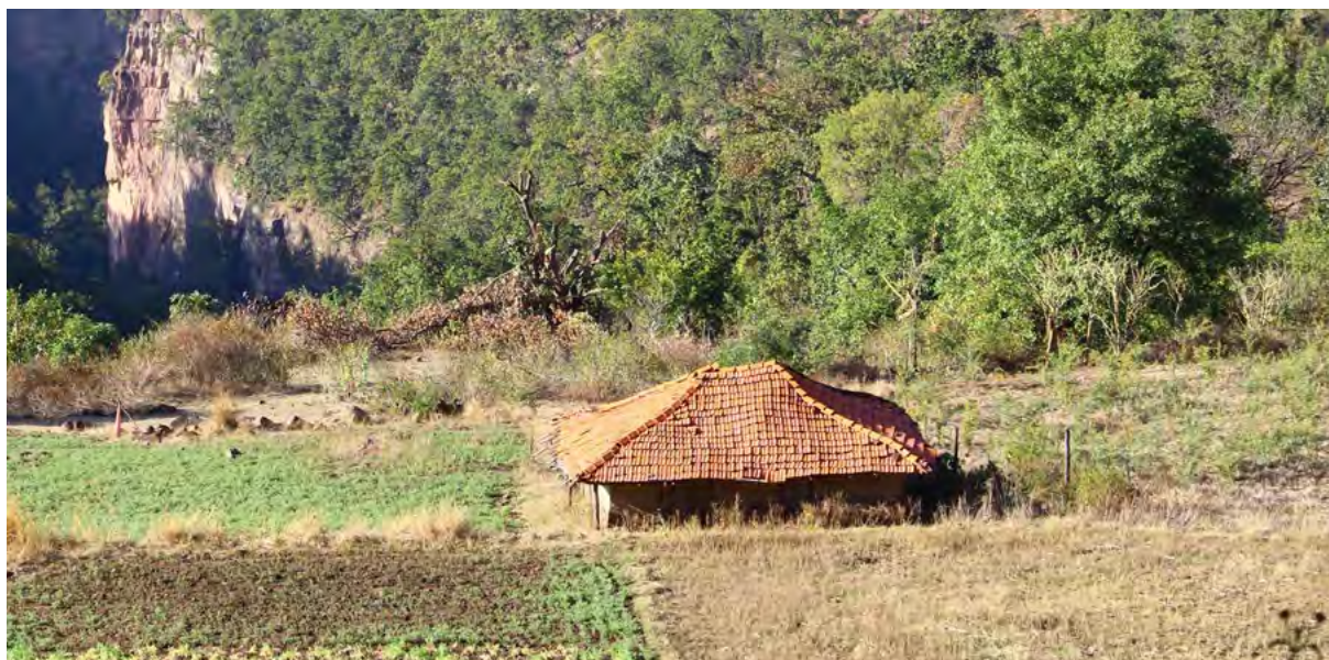
Figure 7: Houses in Patalkot are mostly tiled and built of mud with wooden poles | Source: Sunny, 2023
